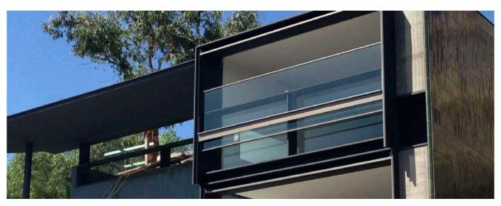
External screens are an aletrnative based on either the Guillotine Glazing or Vertical Motorised system. The latter is a popular selection in the modern environment, with smooth seamless automation; whereas, the Rail system is especially durable in bad weather conditions and affords a solution when an ease of movement is favoured - a simple rail system fits into the pergola's framework systems.
